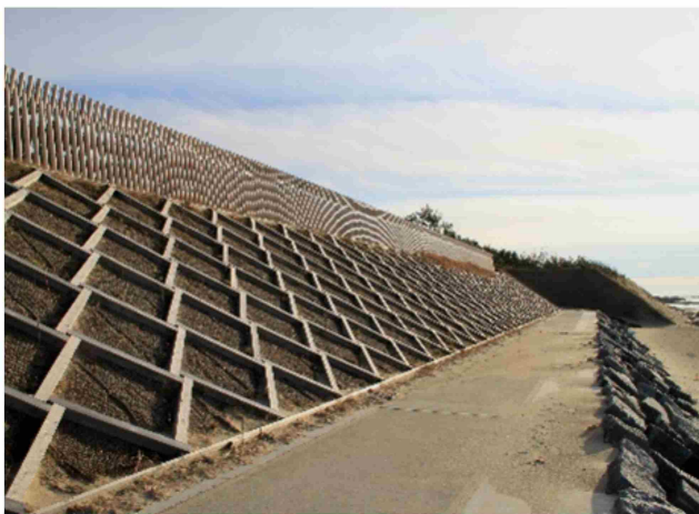
▲ 護岸工と防風柵工の完成
