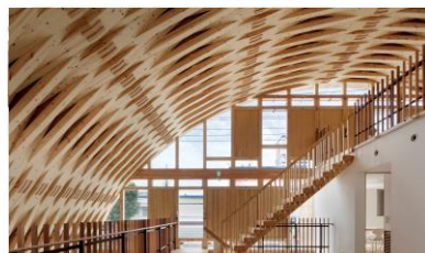
Salon for Housing and Life (Saitama Prefecture) AQURAHOME CO.,LTD., Holzstr Inc., Taiji Kawano Architects, Shinohara Shoten Co., Ltd /Architecture and Space Japan's first medium-sized three-story wooden building constructed with generic lumber and generic processing/construction technologies.
