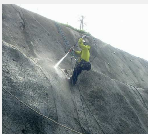
①法面清掃工
